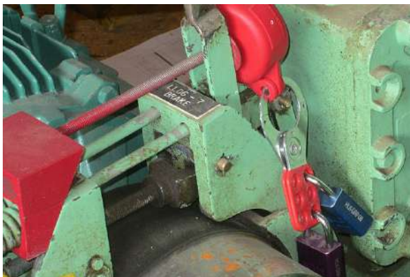
Switches and lockouts
